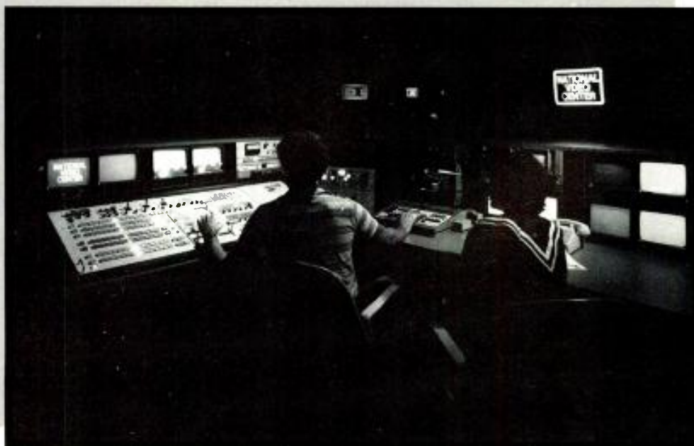
New facility of National Video Center, New York, has edit board in front of operator, switching and other controls close at left.
