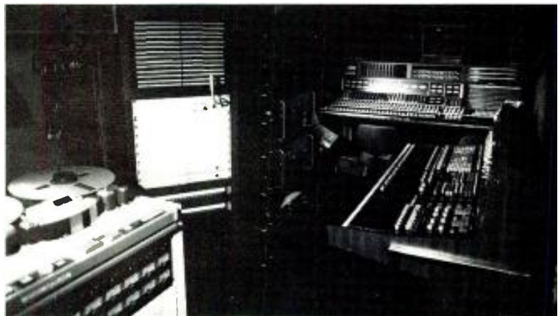
The control room of WGBH's Unit 4 audio control facility features a custom 40x24 API mixing system that provides simultaneous 24-track, stereo, and mono mixes. Outboard equipment includes eight dbx 903 compressor/limiters, dbx 162 stereo program compressor, Lexicon 224 digital reverb system, and two Lexicon PCM 41 DDL effects units. Otari MTR-90 24-track recorder is seen in foreground.
